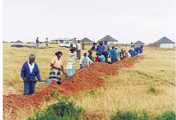
Pipe Trench Being Constructed By Local Villagers
