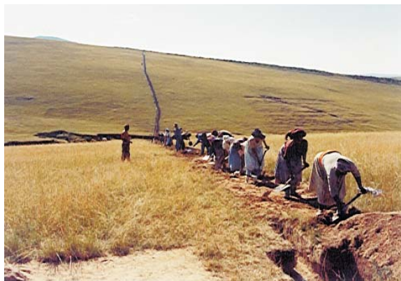
Villagers Laying Pipes
