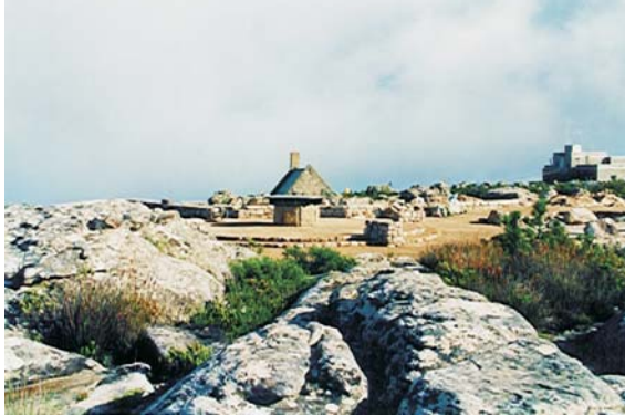
The New Pathways over the Top of the Underground Reservoir
