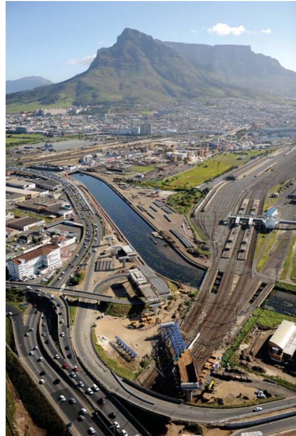
70 m insitu box deck span over railway line shown in clear relief in the aerial photograph
