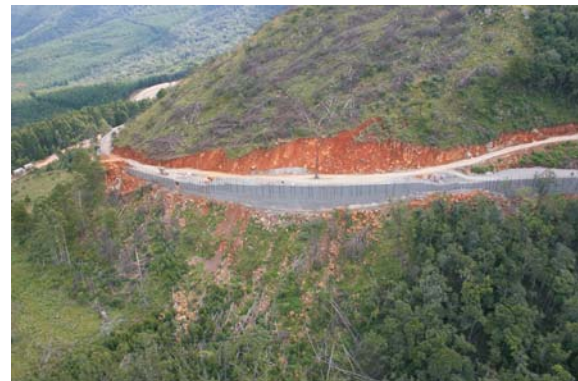
Partially completed earth reinforced & soil nailed wall
