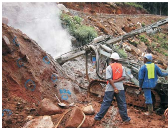
Drilling in soil nails
