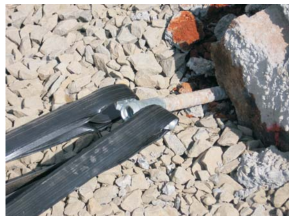
Connection of paraweb straps to soil nail heads
