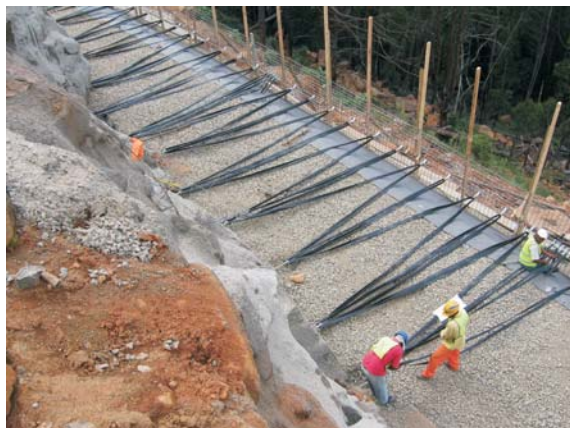
Polyester straps linking mesh facing panels with soil nails
