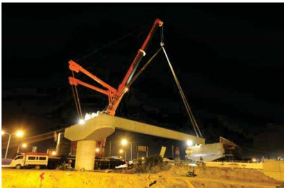
40m long precast beams launched at night to minimise traffic disruption
