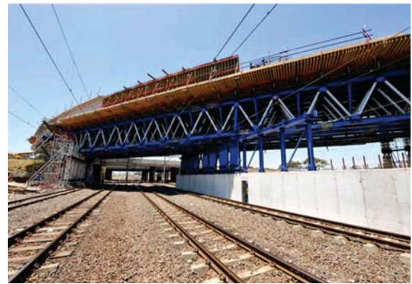
Huge trusses temporarily support the 67 m span across the 8 rail reserve
