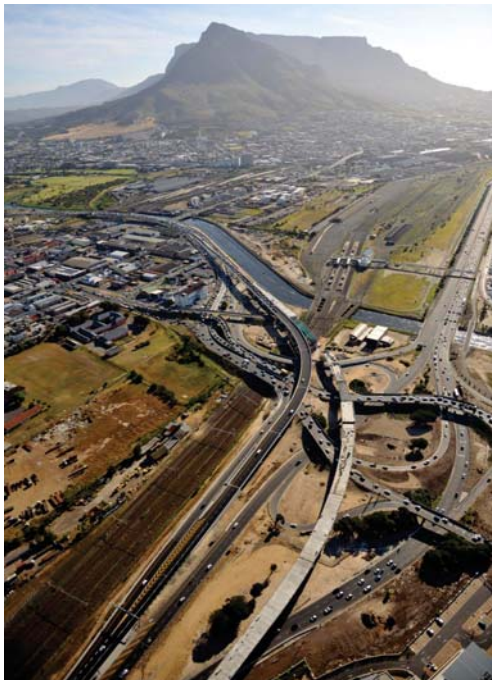
Ramp A completed and operational in time for the World Cup July 2010
