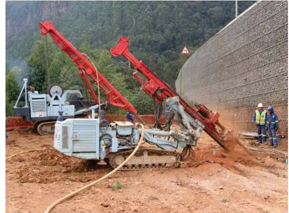
Installation Of Inclined Micropiles Below Existing Retaining Wall
