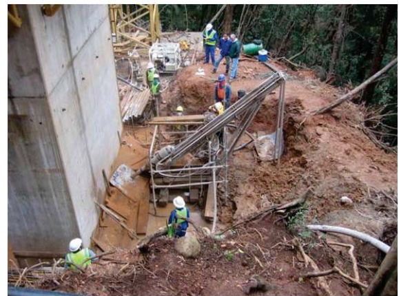
Anchoring Spread Footing Of A Viaduct Into Rock
