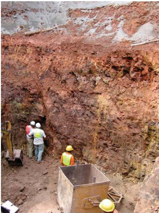
Mapping Geological Structure In A Foundation Excavation
