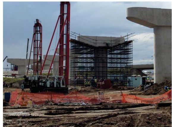
Pile Installation At Koeberg Interchange
