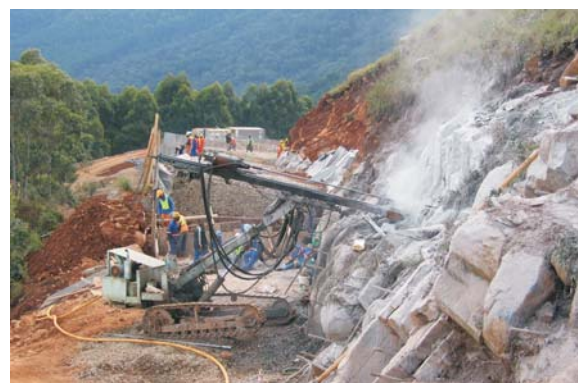
Terranail installation in talus
