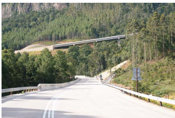
Viaduct 1 & concrete road
