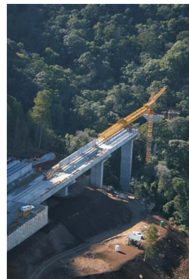
Viaduct under construction
