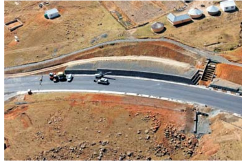
Nyibeni Village gabion toe berm
