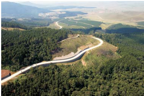
Reinforced earth and gabion retaining walls with sawmill in background
