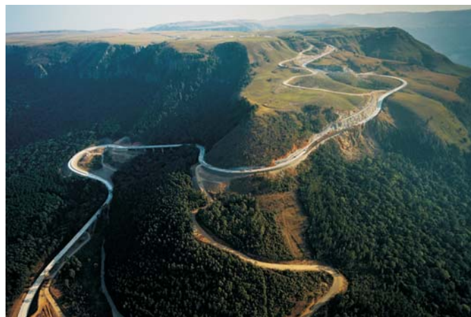
Completed mountain pass
